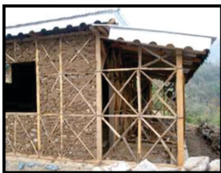
Figure 3: A typical Dhajji Walls
